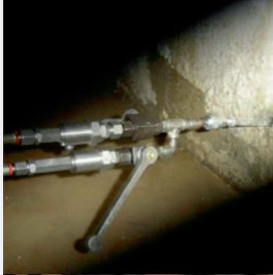
2 component injection head with static mixer
